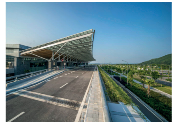
© Van Don International Airport
