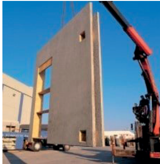
Fig.1. Precast Flat Panel System
