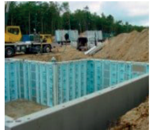
Fig.4. Precast Concrete Foundations
